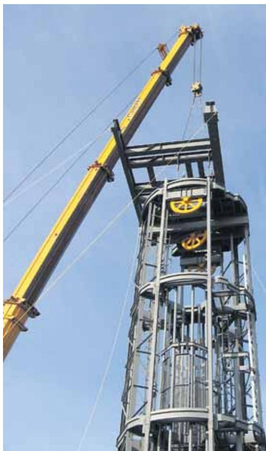
A crane lowers a galloway, a working platform that can have several working decks, into a mine shaft to continue the sinking process.
